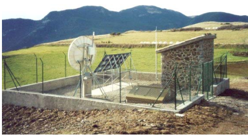
Fig. 2. View of VSAT- Bruguera Station
