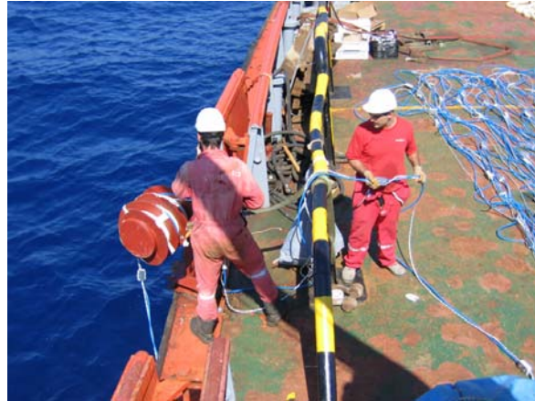
Figure 3: Cables' launching, once jointed with ballasts.
