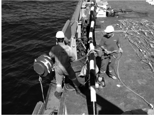
Figure 3: Cables' launching once jointed with ballasts.
