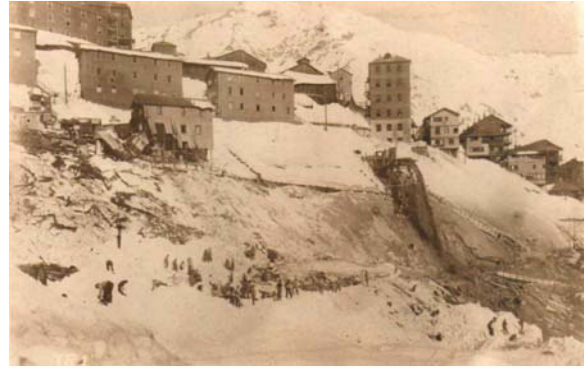
Figure 3. Damages on buildings and Rebolledo Bridge caused by the avalanche of 1941 (source: Sewell Museum).
