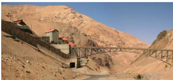
Figure 6. Rebolledo bridge current situation and protection dikes for Sewell.
