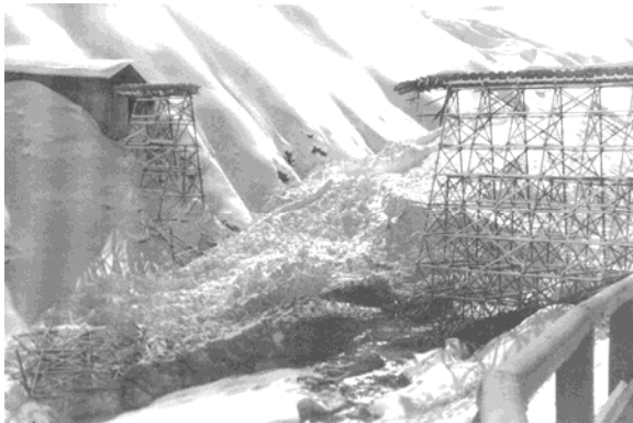
Figure 2. Run-out of the 1926 avalanche, damaging the old Rebolledo Bridge (source: Sewell Museum).
