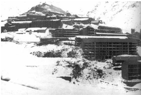
Figure 5. Damages on buildings caused by the avalanche of 1944 (source: León, 2003).
