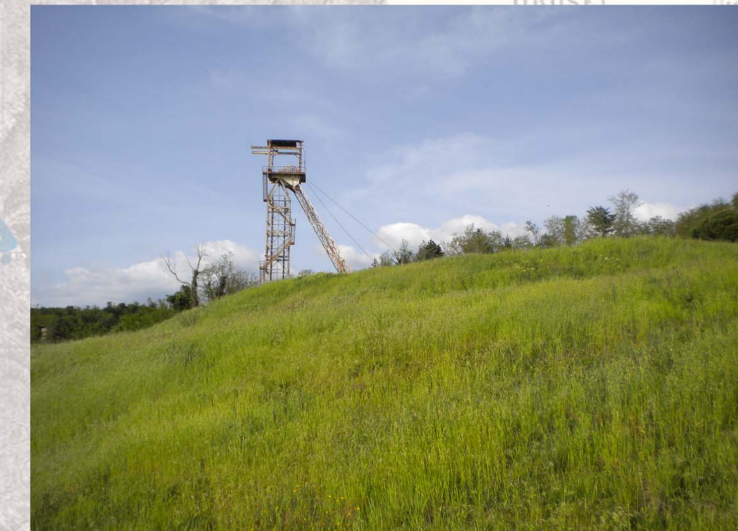
Mining area of Niccioletta: Pozzo Rostan with reclaimed landfill below
