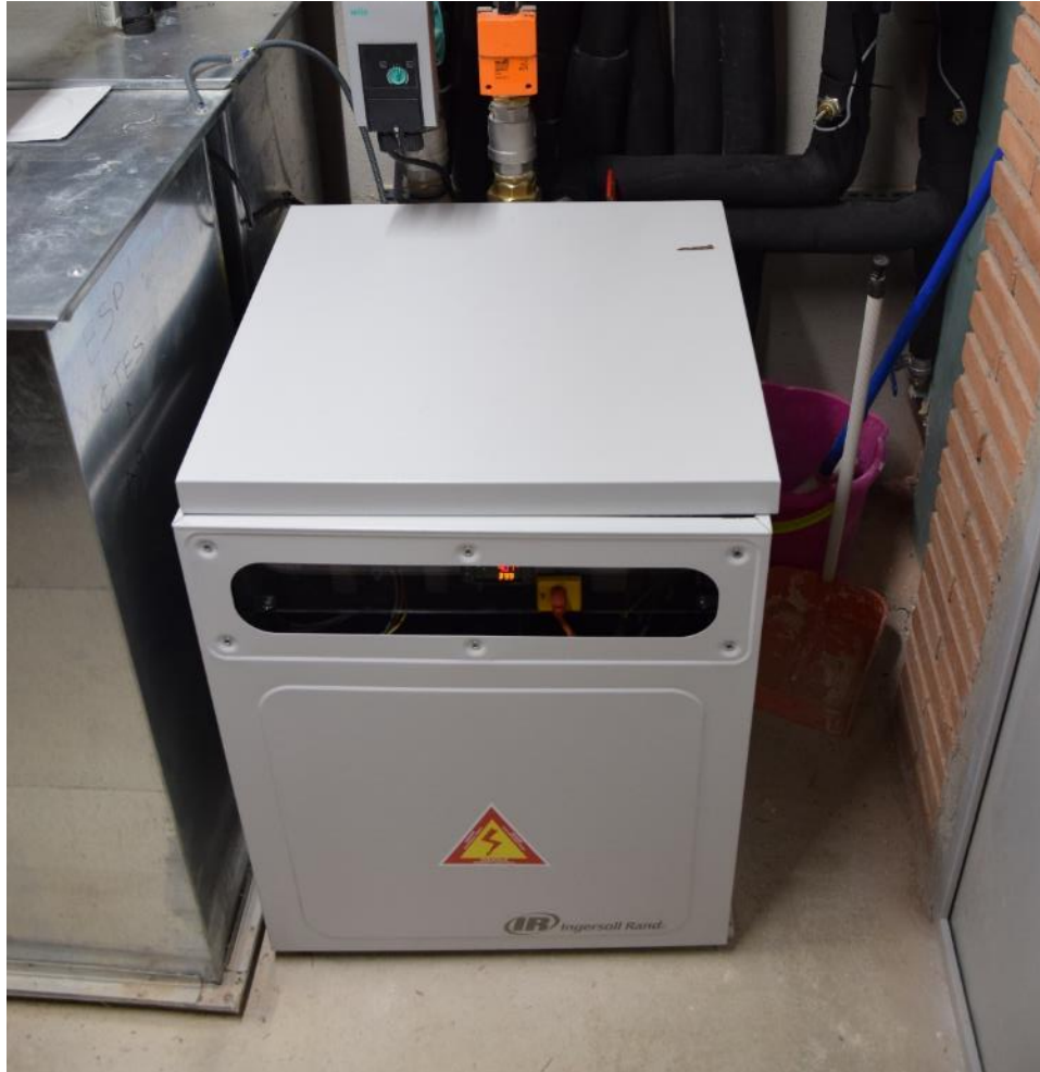
GSHP: 14KW – Heating-Cooling - DHW
